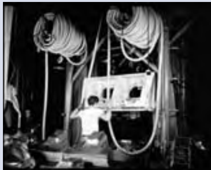
Heavy hemp rope was used to manufacture metal parts for bombers and fighters in 1942 at an aviation plant in Inglewood, Calif. Photo by Alfred Palmer, Office of War Information Collection.
