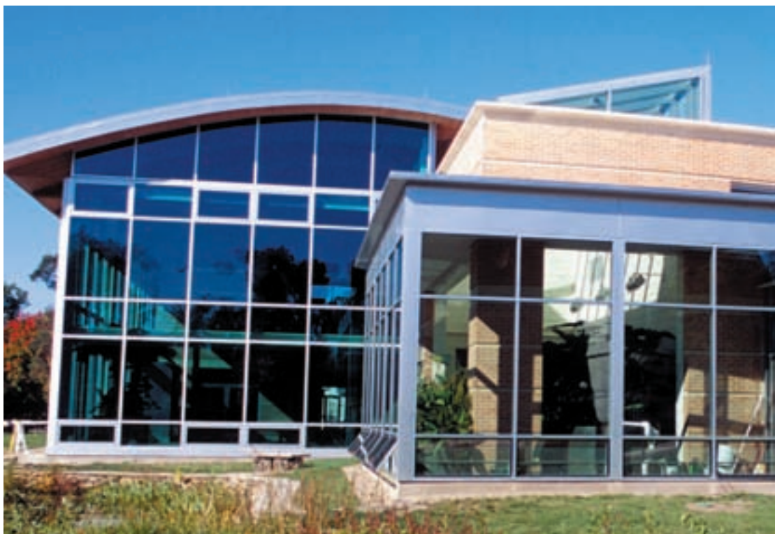
The Adam Joseph Lewis Center for Environmental Studies at Oberlin College is a "living machine" that combines elements of conventional wastewater technology with the purification processes of natural wetland ecosystems to treat and then recycle the building's water.
