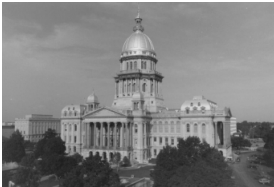
Security at public buildings such as the Illinois Capitol has become a priority issue in recent months. (Photo: state of Illinois)
